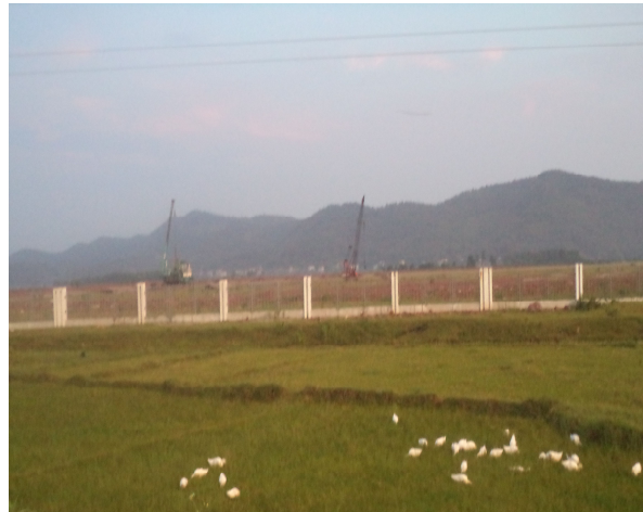
Van Trung Industrial Zone after 5 years implementation
